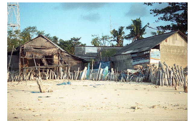
Temporary seawall on Nusa Lembongan made from sticks and coral. Source: Catherine Kerr
