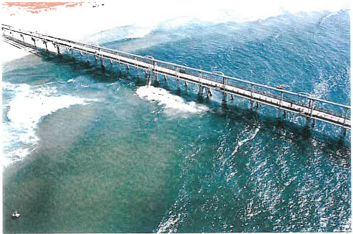
Plate 8 : Aerial view of the turbid plume from jet pump no. 3. The distance of travel of the plume is illustrated by the 10m separation between the supporting piles of the jetty.
